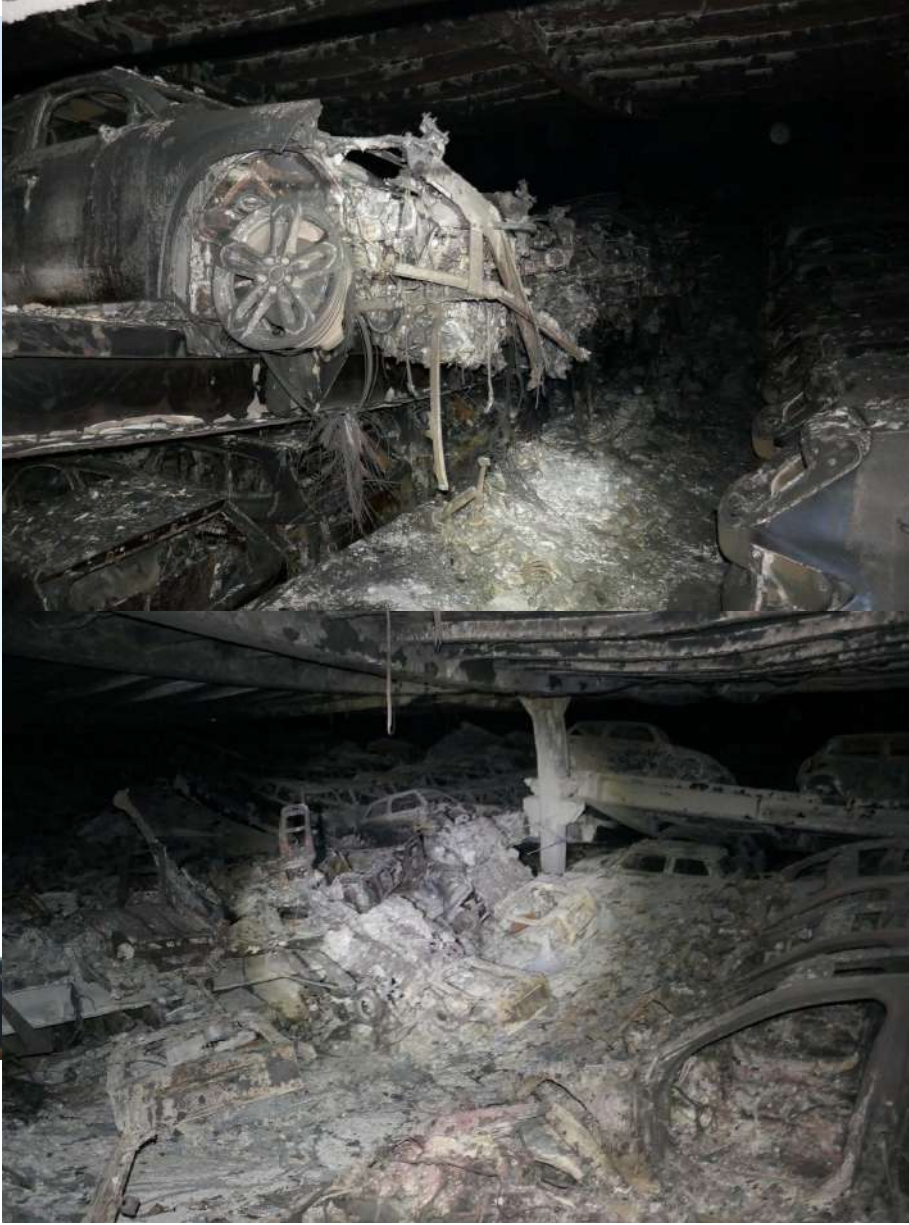
Structural damage to internal and external items resulting in displacement and failure of decks.
