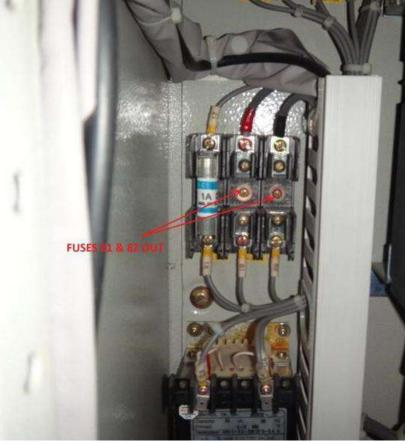
Two fuses of the circuit were removed
